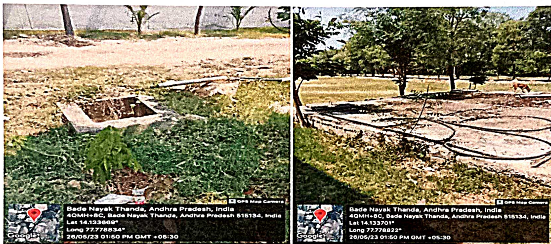
Fig-7: Rain water which is collected from the roof top of the buildings is stored in the rain water harvesting pits and a huge sump.
